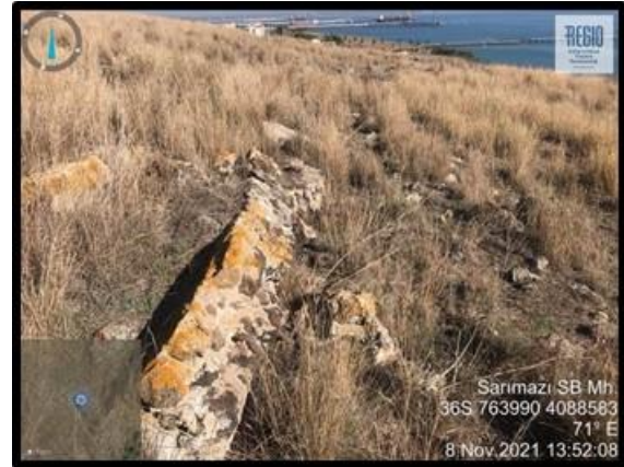
Figure 5-5. Kurtpınar Ancient Waterway Mortared Wall
